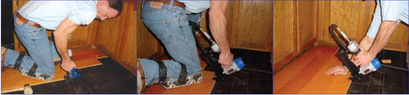
These three photos demonstrate the HIGHPRO tool in action with both a conventional and reverse grip. The reverse grip capability comes in handy for tight quarters.
