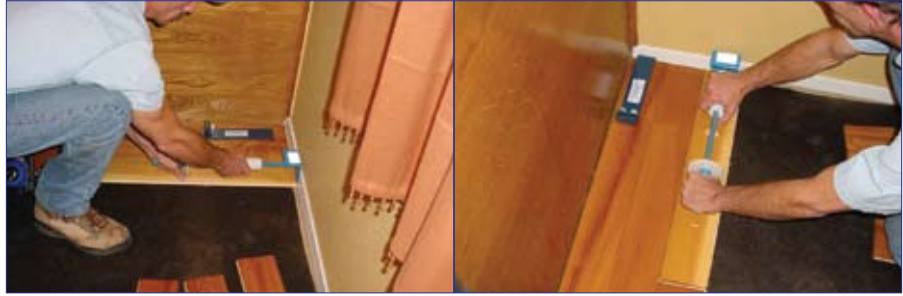
These pictures demonstrate the Lam-Hammer in the field, using it to bring the board in tight.
